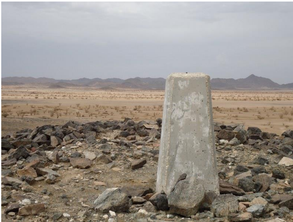
Figure 11: Geodetic pillar type 1
